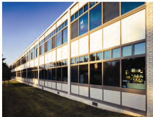
Sycamore Avenue Elementary School Bohemia, NY
